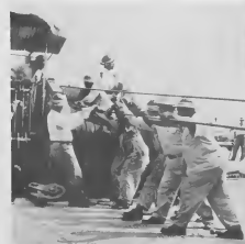
EVERYONE LENDS a hand to straighten out cable on the hoist's bottom drum. At this stage one part could roll over and cut the cable, which has all the load. TIR TA duna un man pa drecha un cable ariba e drum mas aban di e. Na e punto aki un parti por lora over y corta e cable cu ta wanta tur e peso.
